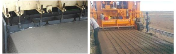
The slipform paver can be designed for different templates according to the user's different road crosssectional shapes to meet the user's pavement shaping requirements.
